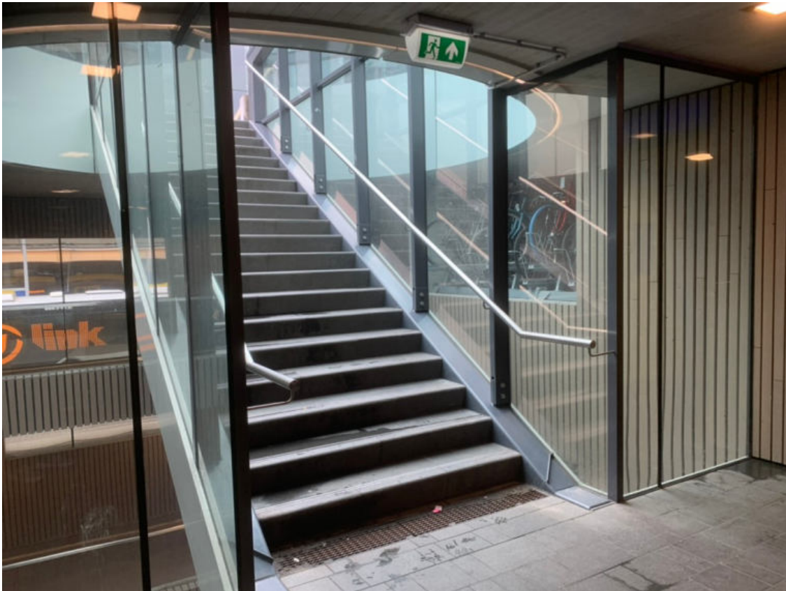
Fig. 30 Pedestrian exit from inside the facility (15.05.2023, Henrike Kramer, Utrecht)
